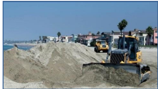
Figure 10. Sand berms being made along the Long Beach Peninsula in preparation of high surf. Photograph by Chris Carlson (AP 2014)
